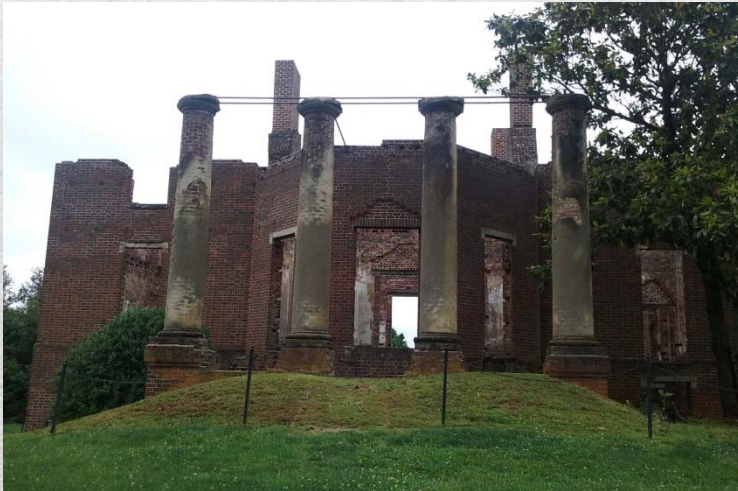
Barboursville mansion. Stabilized ruins.
