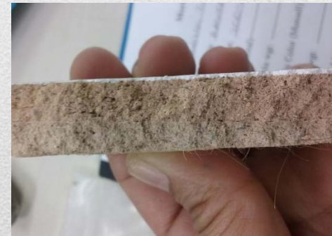
Rivermount House’s plaster sample.
