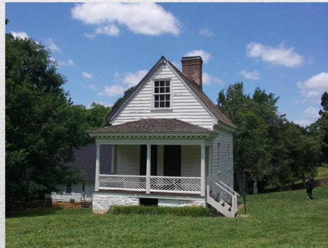
Preswold Plantation. Office, restored and conserved.
