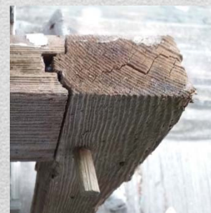
Evidence of sash joined by pegs.
