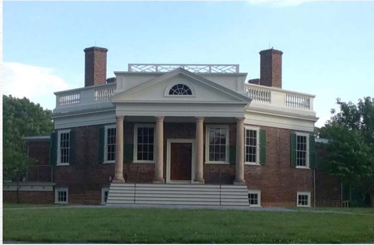
Poplar Forest, on-going restoration project.
