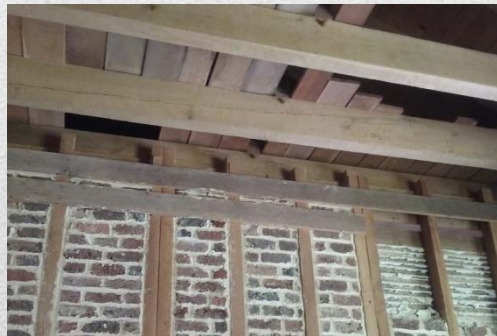
PF interior restoration process.
