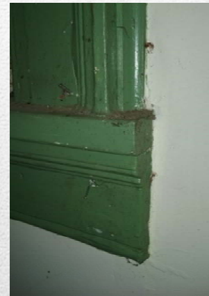
Wood molding survey.
