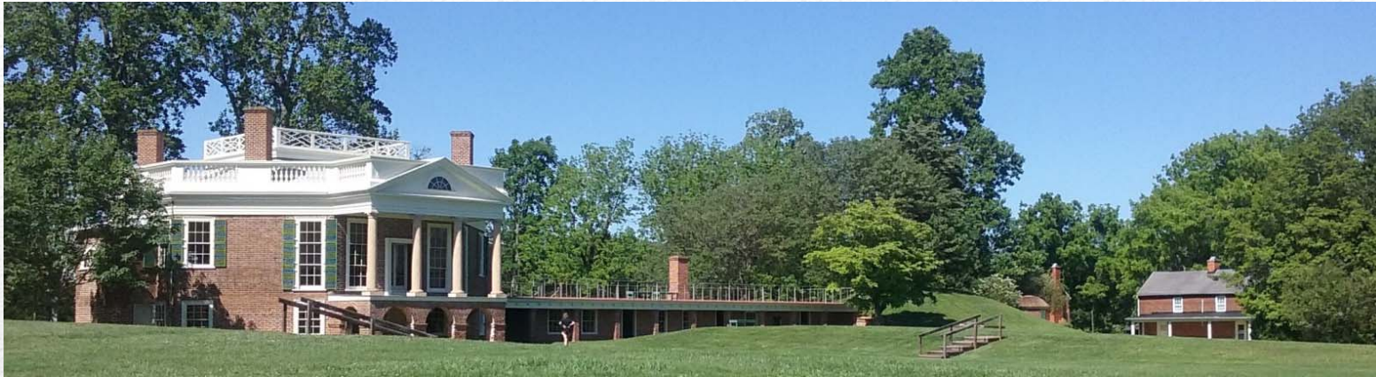
Poplar Forest's south façade, wing of offices, lawn, and slaves' house.
